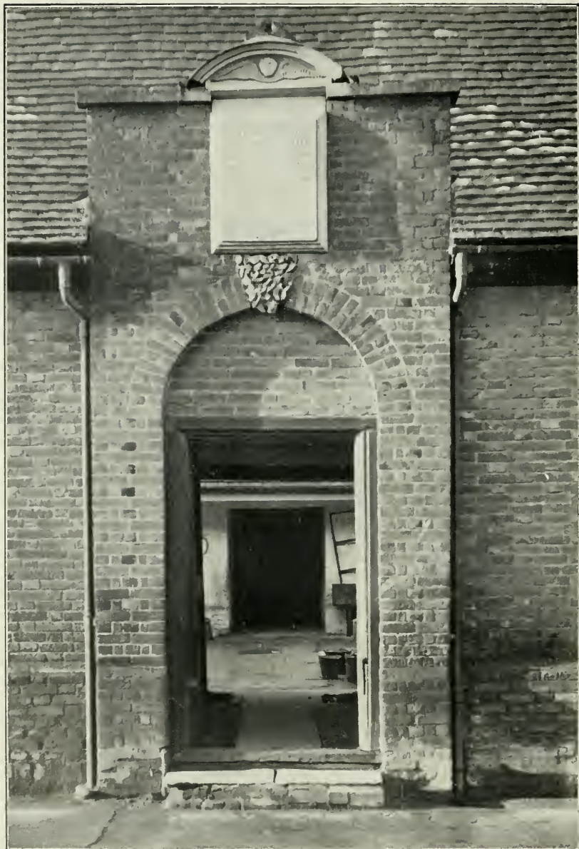
ENTRANCE TO STILES ALMSHOUSES, WANTAGE.
